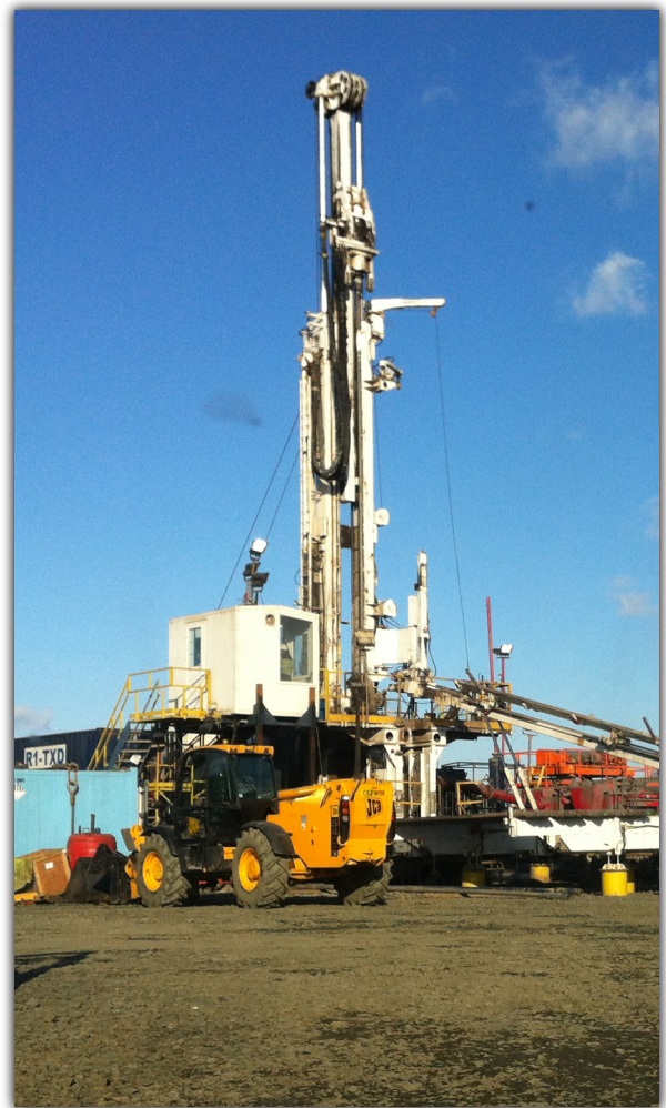
CSG/CBM rig used on project in Central Scotland
